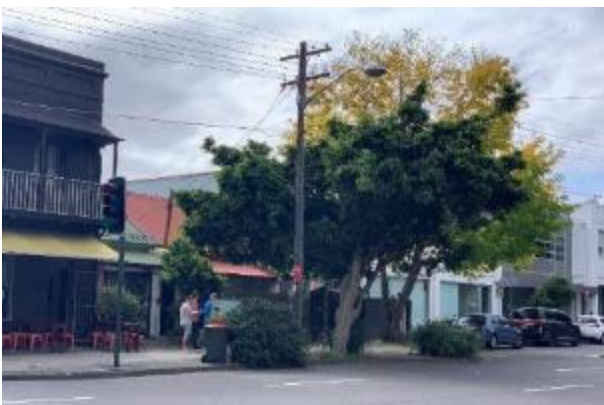
Figure 26. 88, 86, 84, 82, 80 and 44-78 Rosehill Street, Redfern
