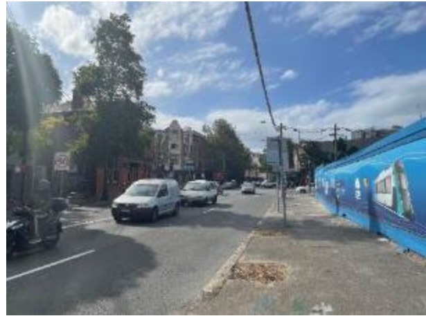
Figure 11. Future Waterloo Metro Station, 56-58 and 60 Botany Road, Alexandria
