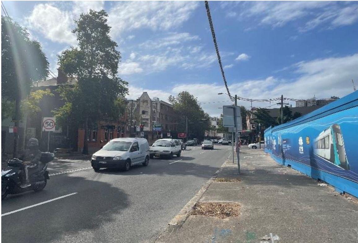
Figure 5: Future Waterloo Metro Station, looking west
