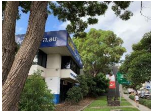
Figure 15. 216-220 Wyndham Street, Alexandria, looking east at the SP2 setback on McEvoy Street
