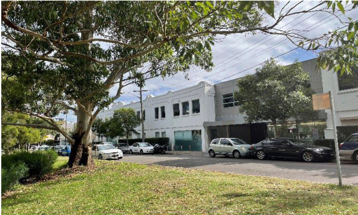
Figure 7: 44-78 Rosehill Street, Alexandria, looking west
